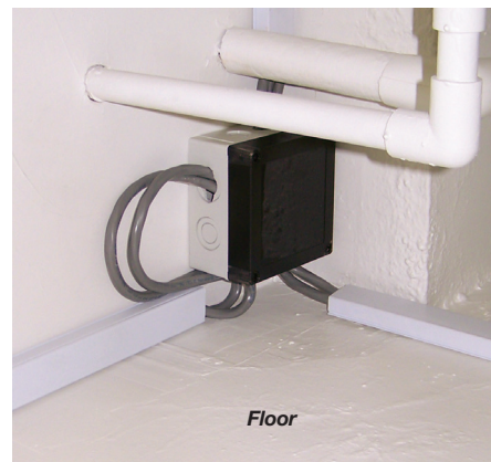
Wall-mounted coils are a practical alternative to column and floor-mounted coils for TEMs and SEMs installed near the center of a room.
