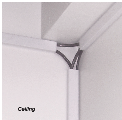
Wall-mounted coils are a practical alternative to column and floor-mounted coils for TEMs and SEMs installed near the center of a room.
